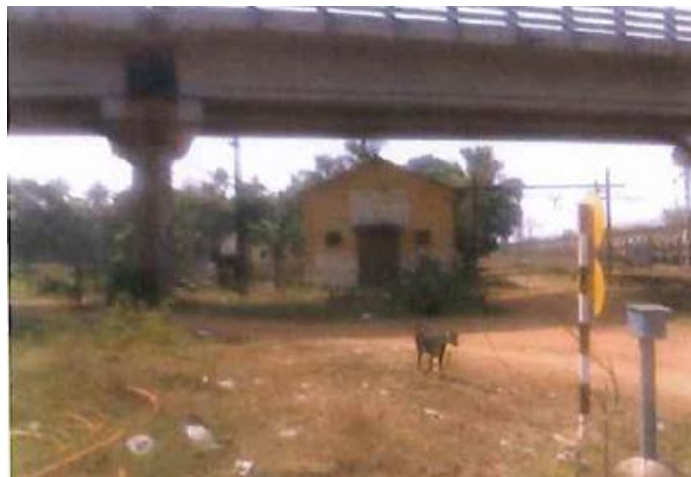
Figure 13 View from TP-16 towards TP-17 under the bridge.
