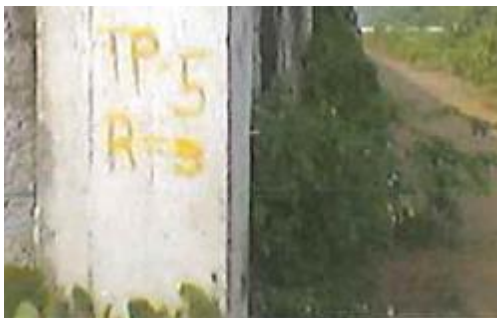
(a)View from TP-05 towards TP-04
