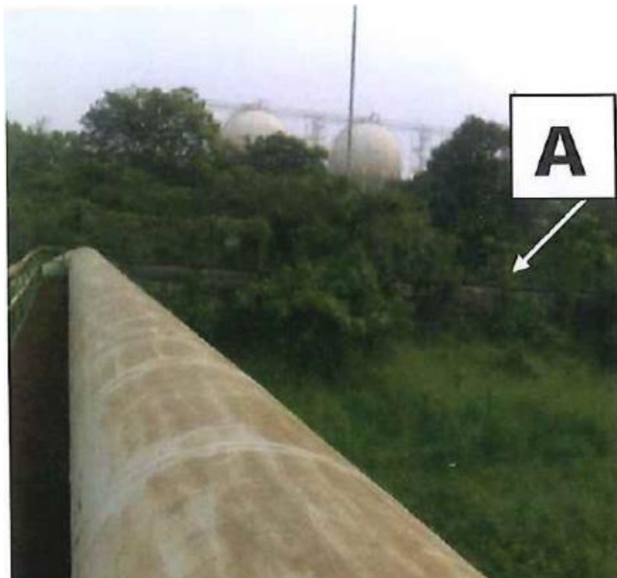
Figure 1 View from TP-01 to TP-00
