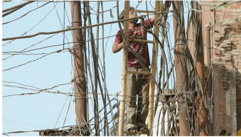
Figure 4.3: Electricity Stealing or in local Katiya in Kanpur city
