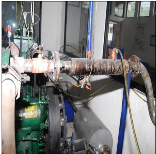
Figure AE.4 Heat exchanger
