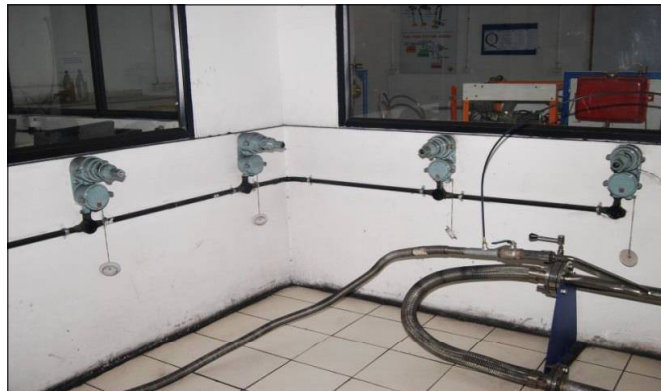
Figure AE.11 Switches
