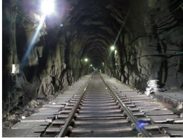
Fig. 6.3 Railway tunnel carved through hard rock
