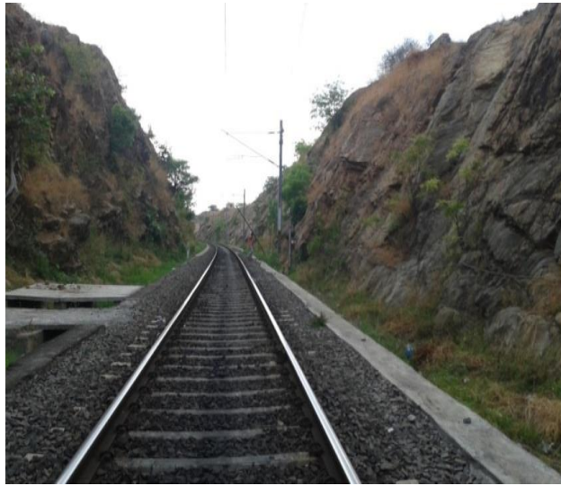
Fig. 4.2 Electrified track through the earth cutting
