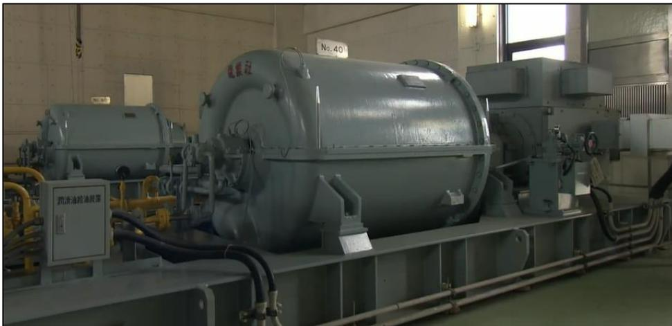
**Figure 5.1:** The ventilator used to provide aeration in a wastewater treatment plant in Yokohama, Japan. Based on the data sheet from the plant, the ventilator units that sends in oxygen to the aeration tank alone consumes 40% of the total energy consumption by the plant. (Source: Environmental Planning Bureau, Yokohama, Japan).
