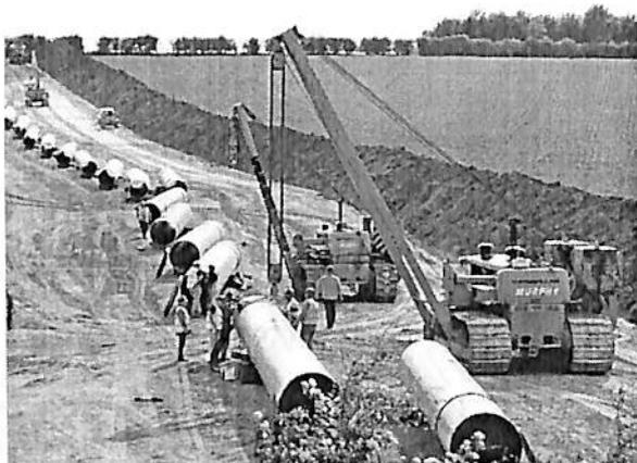
Figure 5: Transco X80 pipeline construction
