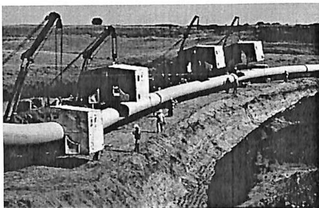
Figure 4: construction of X80 line pipe
